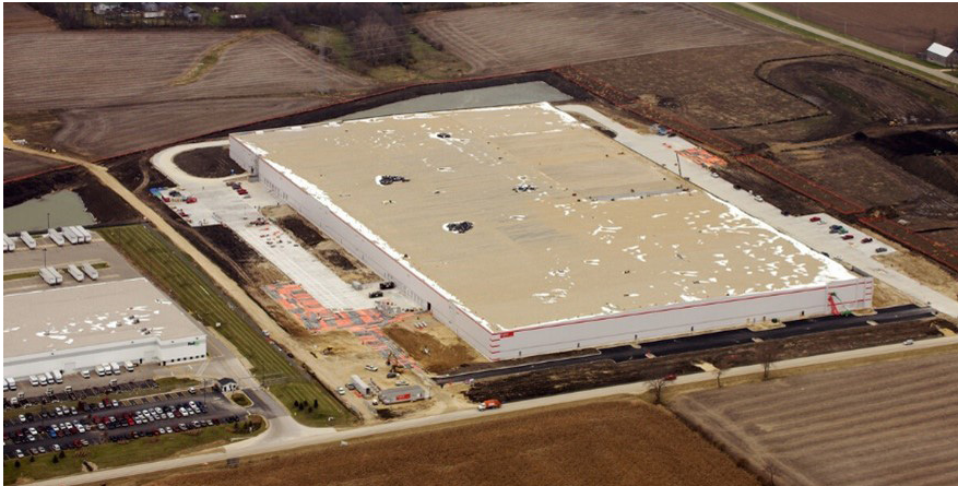
Work in progress on Berner's state-of-the-art 675,000 SF specialized production/distribution facility.
